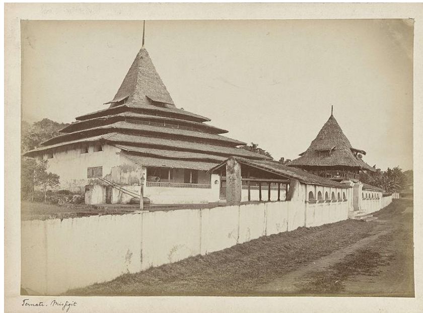
Figure 10: Masjid (mosque) Sultan of Ternate Mosque (Indonesian Masjid Sultan Ternate), also known as the Old Mosque of Ternate, is an old mosque in Ternate City, Indonesia is an example of the typical pyramidal multi-roofed timber structure (Source: Darmayanti and Bahauddin 2015).
