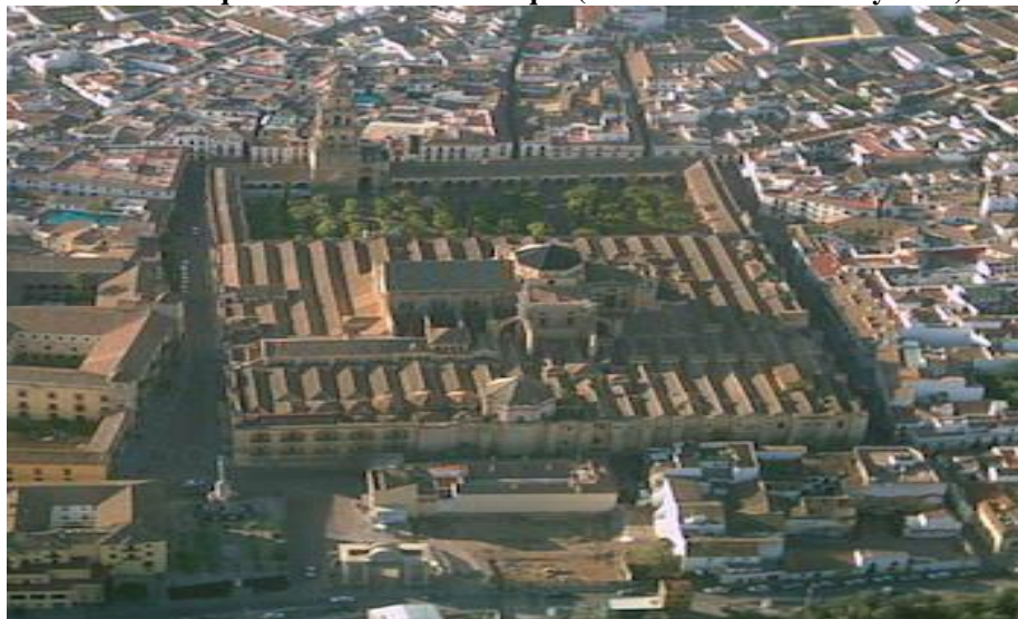
Figure 6: An aerial view of the Great Mosque, Cordoba, shows its remarkable roof structure of gables as an example of the hypostyle structure (Source: The Great Mosque of Cordoba (article) Khan Academy 2018).
