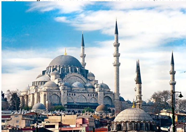
Figure 8: The Suleymaniye Mosque, Istanbul, one of many splendid examples of massive central dome surrounded and supported by two half domes, rests on four pillars. It is one of the most ambitious work of architect Sinan (Source: Numan and Santosa 2018).
