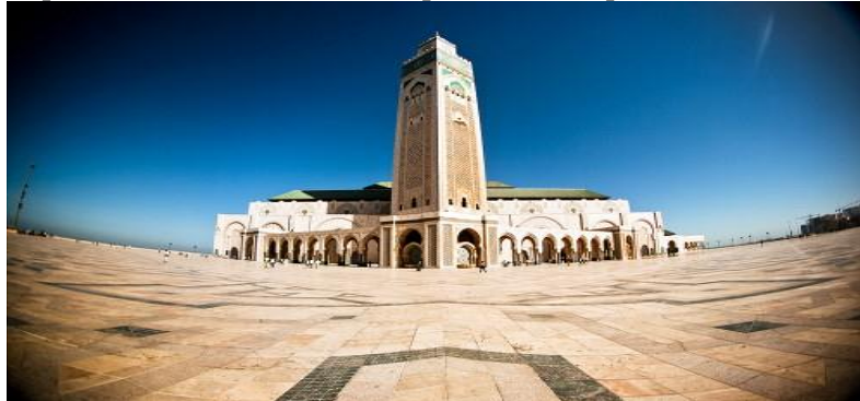
Figure 15: King Hassan II mosque in Casablanca, Morocco (Source: El Guabli 2018).
