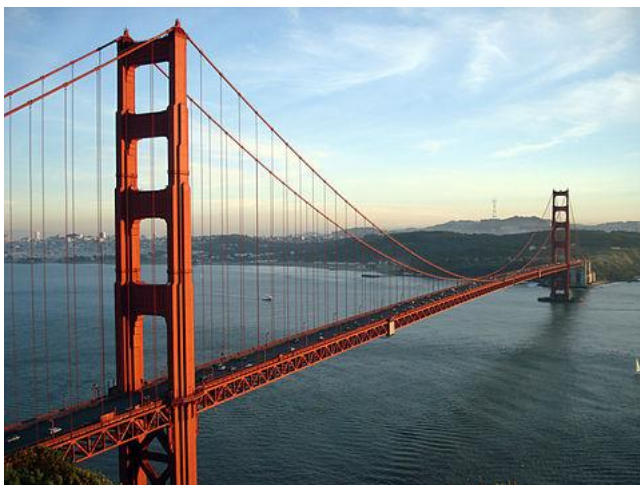
Figure 7 Golden Gate Bridge (USA, 1937)
