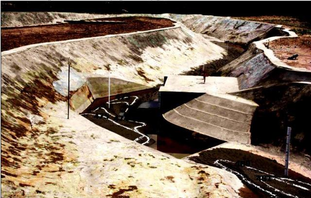
Fig. 7b. Riverbed Sediment Profile downstream after flushing
