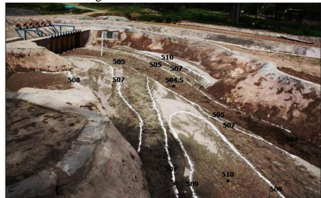
**Fig. 7a. Riverbed Sediment Profile upstream after flushing**
