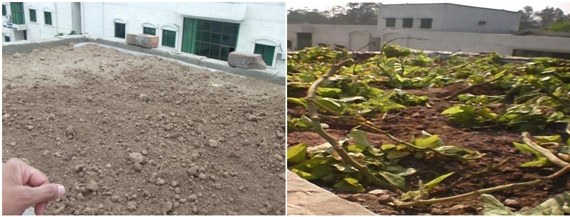
Figure – 3: Various Steps Showing Construction of Green Roof.
